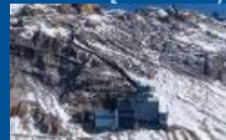
Environmental Research Station Schneefernerhaus Garmisch-Partenkirchen
